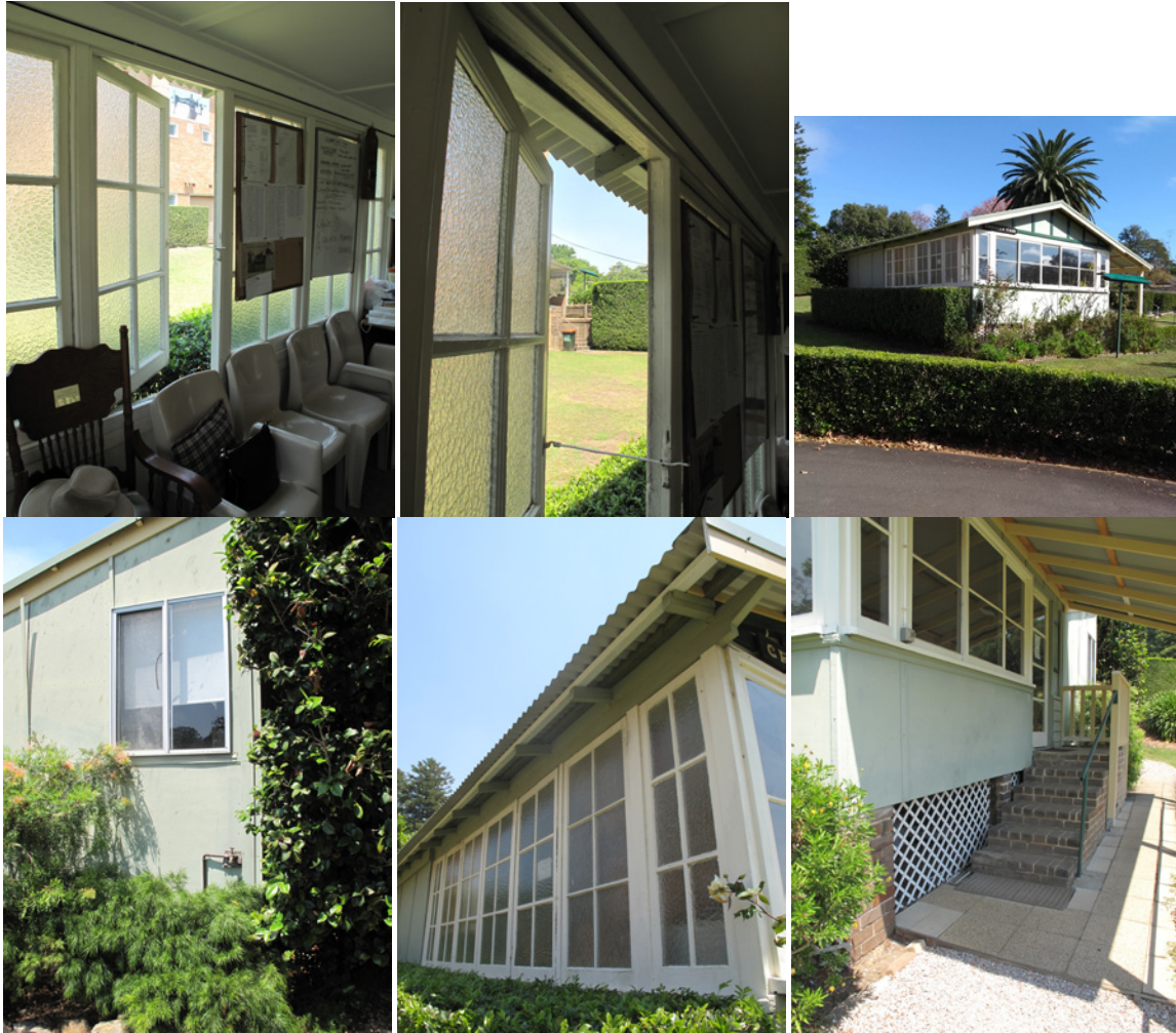
Fig. 6.12 Croquet Clubhouse : Details of Fenestration, Bressumer and Brick Steps (2019) [S. Cremona : SRTC 2019]
