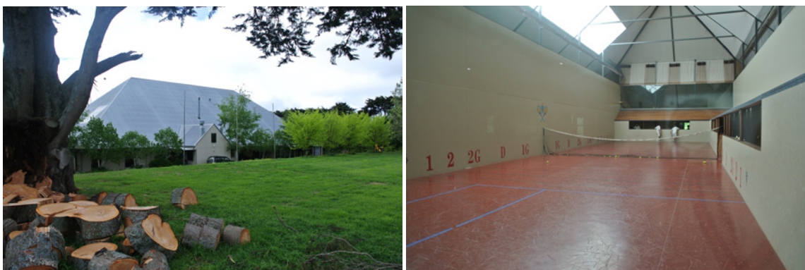
Fig. 2.10 Cope-Williams Real Tennis Court at Romsey, Victoria : Erected 1998 The Main Wall is built of pre-cast concrete panels (LHS) [Collection AFW]
